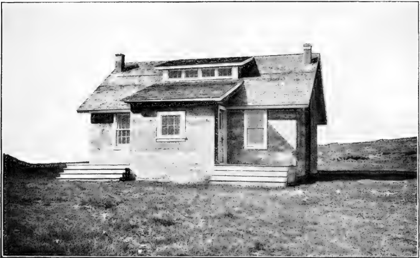
FIG. 14.—TYPE OF CONCRETE HOUSE BEING BUILT ON PRIBILOF ISLANDS FOR NATIVE RESIDENTS.
